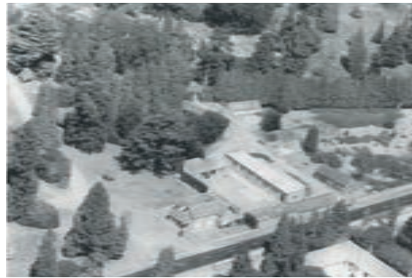
Superintendent's office area including the former masonry works c. 1970
