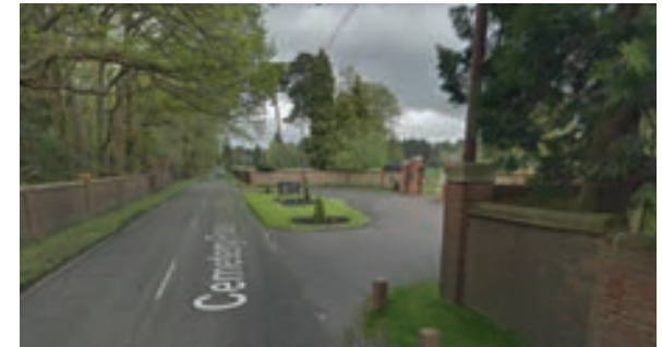
The curved forecourt to the Glades would be mirrored to form an entrance to an area in the north cemetery for a potential new crematorium
