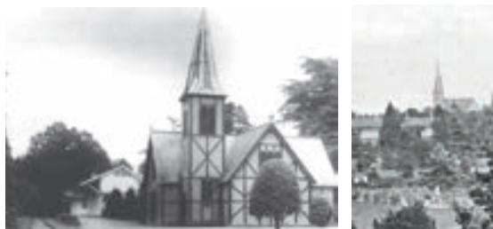
The former south cemetery station
