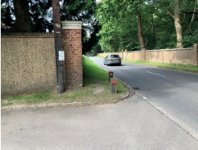
Photograph 2.1: Visibility available from existing access to the left from a 2m setback
