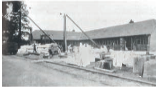
Masonry works building (now Beard Construction HQ)
